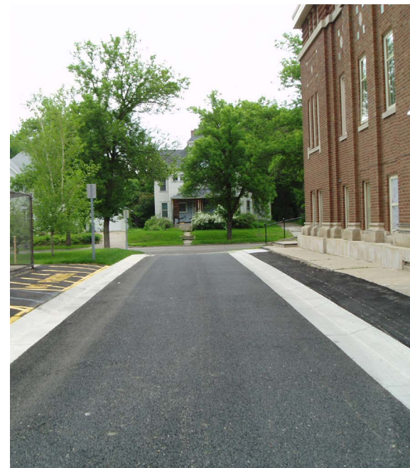
Hamline Green Alley Photo: SRF Consulting Group
